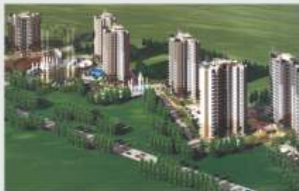
Twin Towers built in 13.5 acre high-rise condominium complex in Sector 57, Gurgaon
